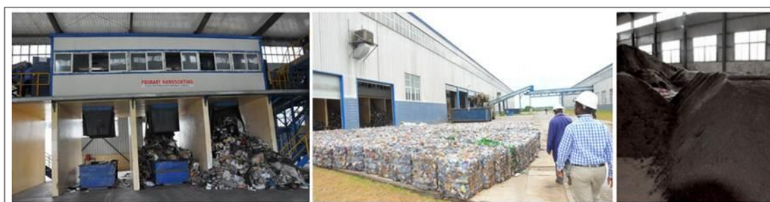
Figure 4.14: Accra Compost & Recycling Plant (ACARP)
