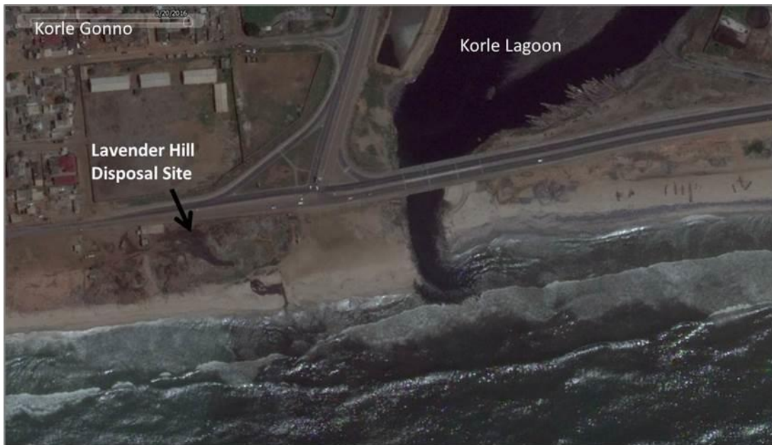
Figure 4.5: Lavender Hill Sewerage Disposal Site
