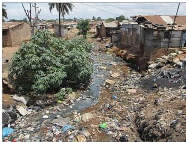
Figure 4.9: Natural Stormwater Channels filled with Solid Waste
