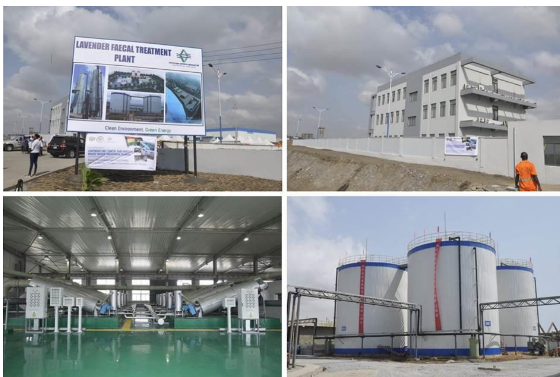
Figure 4.8: Mudor Faecal Treatment Plant
