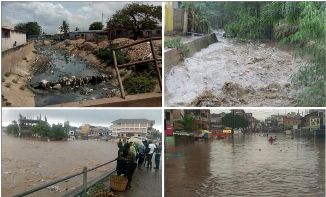
Figure 4.11: Flooding in Accra during 2014 and 2016
